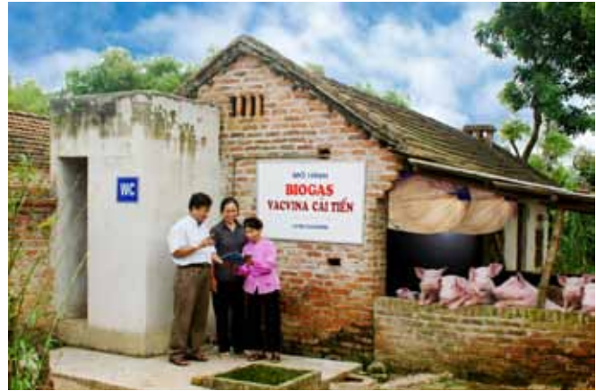
The project site
