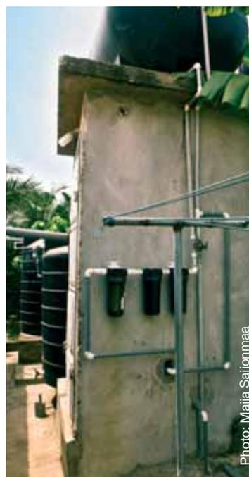
An example of an integrated RWH system with water filters.
